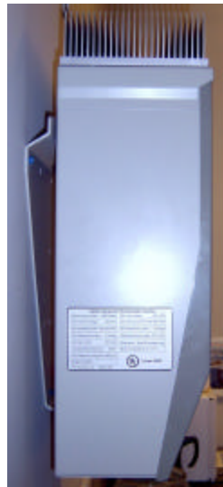
Figure 4: Mounted StarInverter with Mounting Bracket in Place
